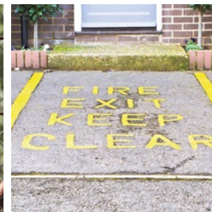
Fire Exit: "No Parking"
